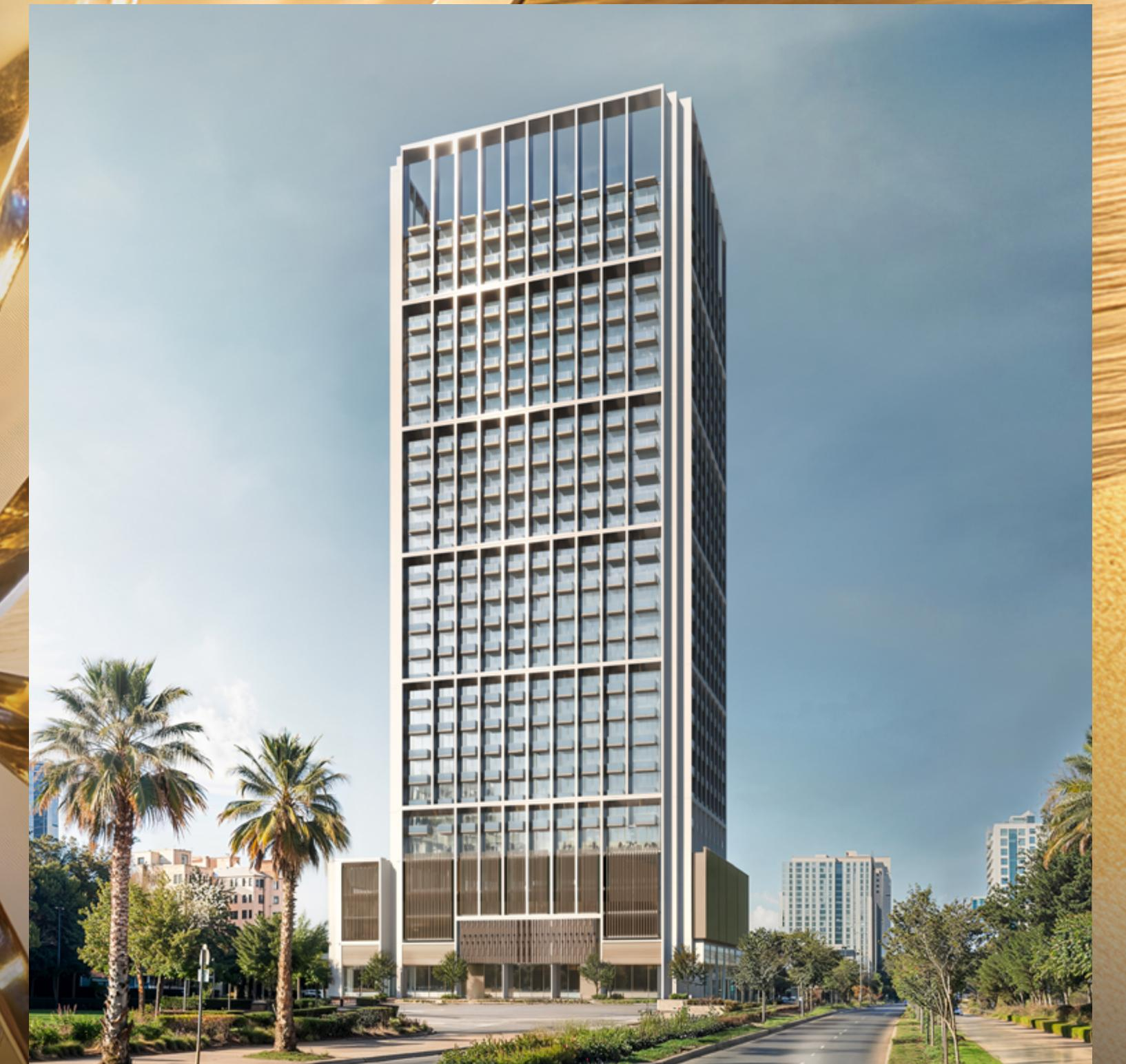
It spans three basements, a ground-floor retail hub and four podium levels. This base supports the 24 residential floors that tower upward, creating a definitive symbol of refined stature.
