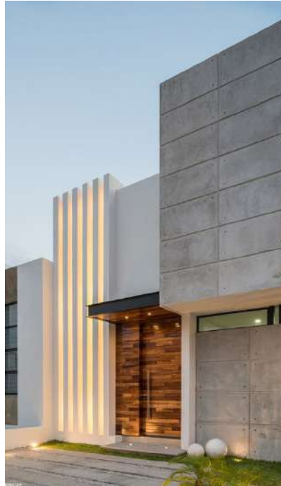
Example of villa lighting
