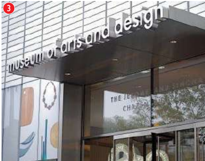
Sign integrated into canopy
