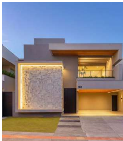
Example of villa lighting
