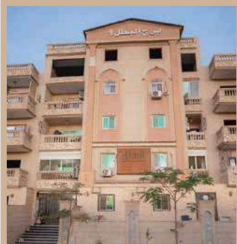
First District Project
