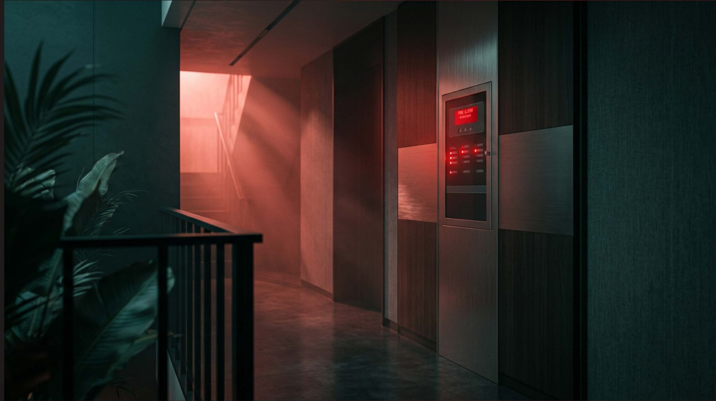
Fire Safety System
